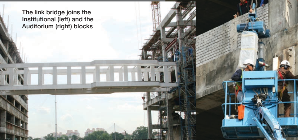
Workmen at level three
