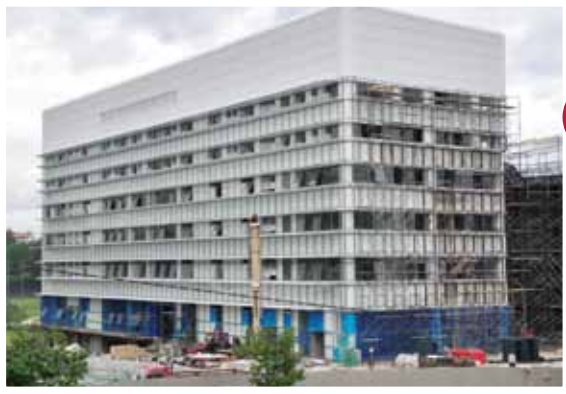
Left: Institutional Block nearing completion
